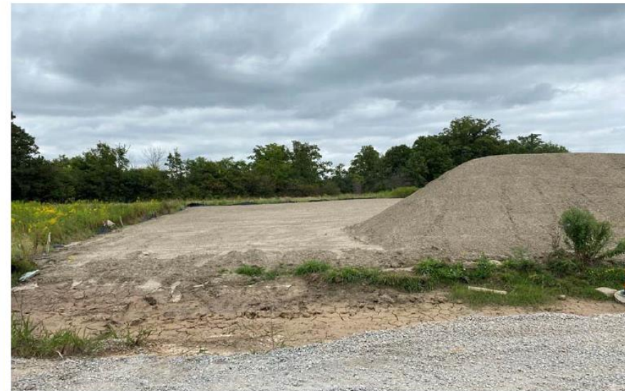
Photo 3. August 29, 2024 - Topsoil temporary staging area
