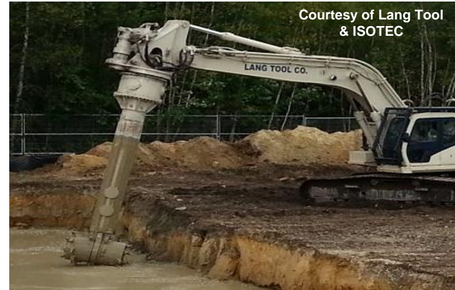
Soil mixing using excavator with dual axis mixing attachment
