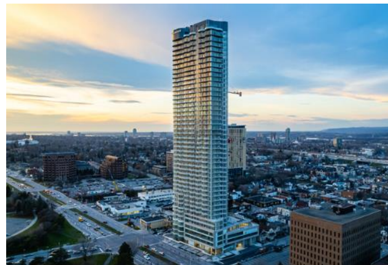
Claridge Icon redevelopment on former Imperial service station property, Ottawa ON
