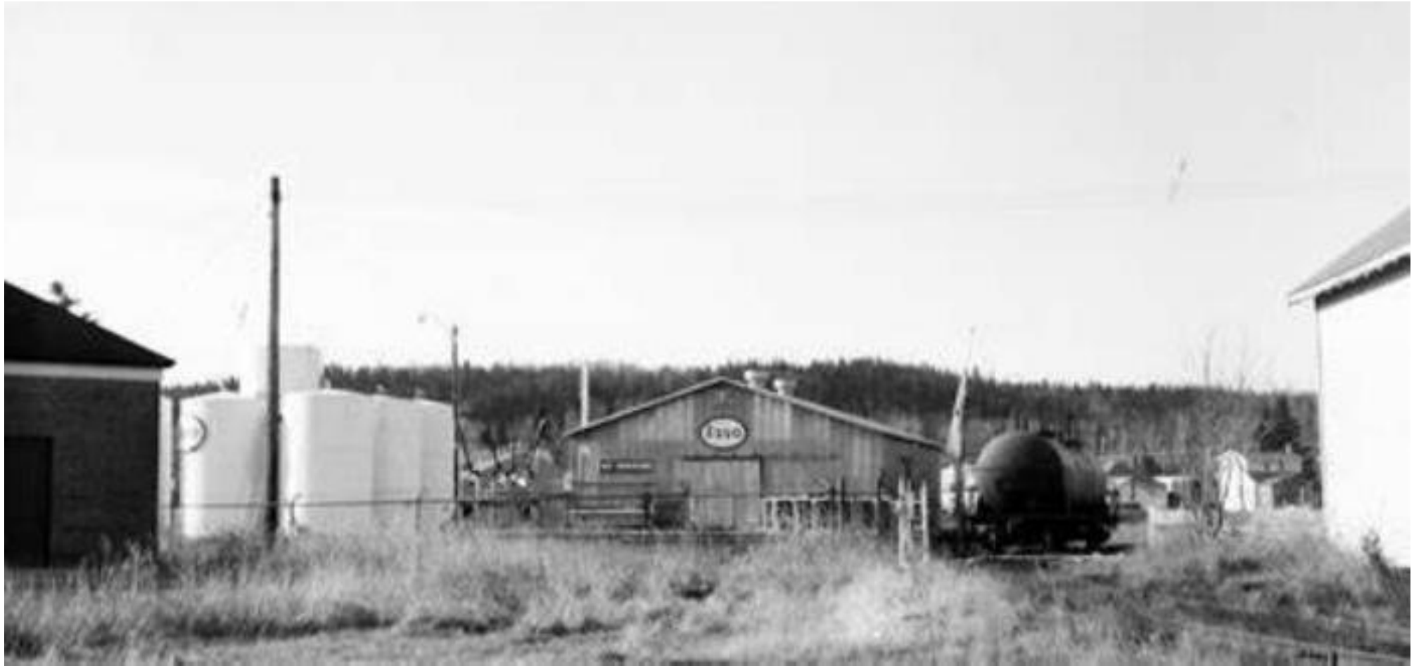
Esso fuel bulk plant with rail supply – 1960s
