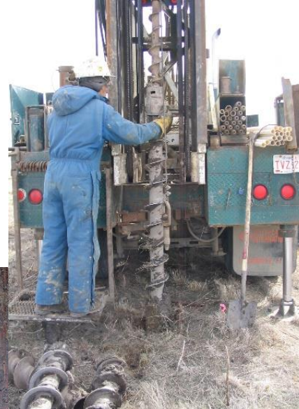
Hollow Stem Drilling
