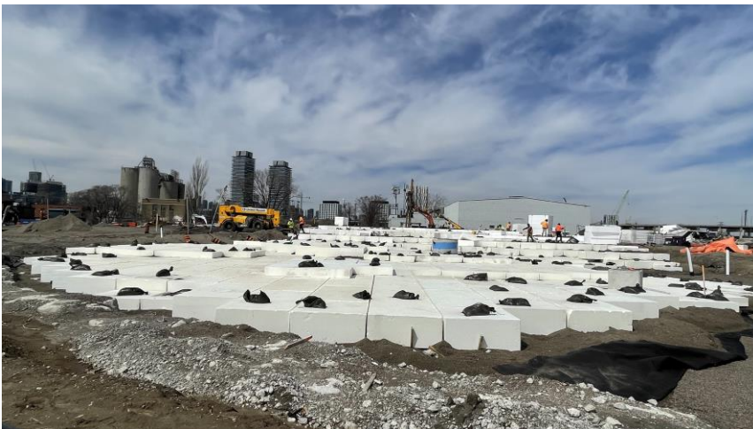
Typical: Lightweight Fill - Transition B 1:7.5
