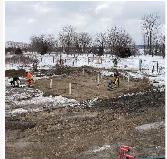
Installing/Compacting of a Low-Permeability Clay Cap
