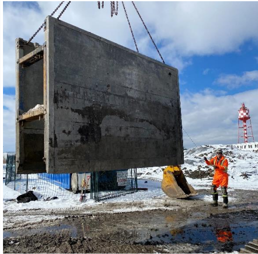
Removing Trench Boxes
