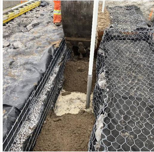
Placing of Pre-Packed Monitoring Wells
