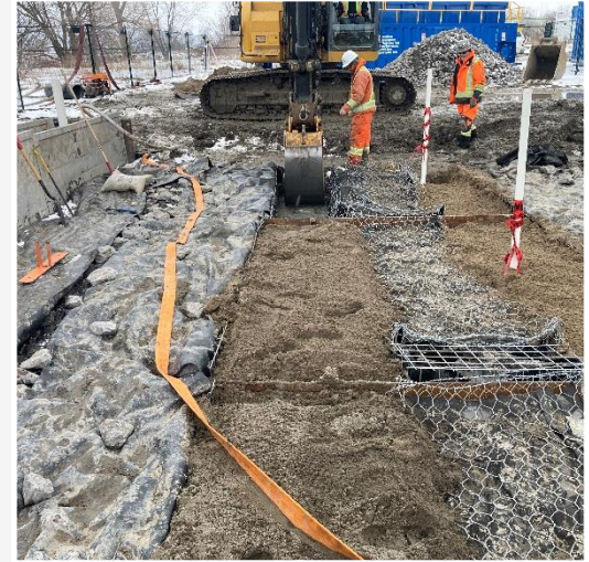
Placing of Adsorption Materials
