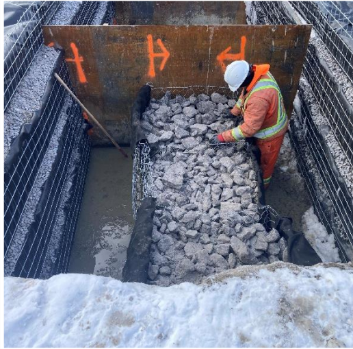
Gabion Partitioning Walls
