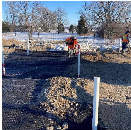
Placing of Granular A on top of Grid and Geotextile layers
