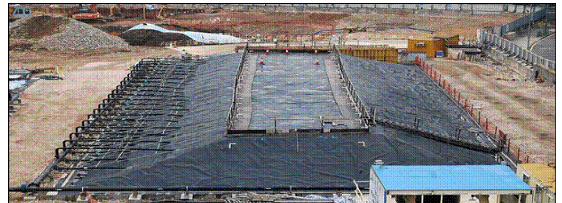
On-site treatment of excavated soil in aerated biopiles
