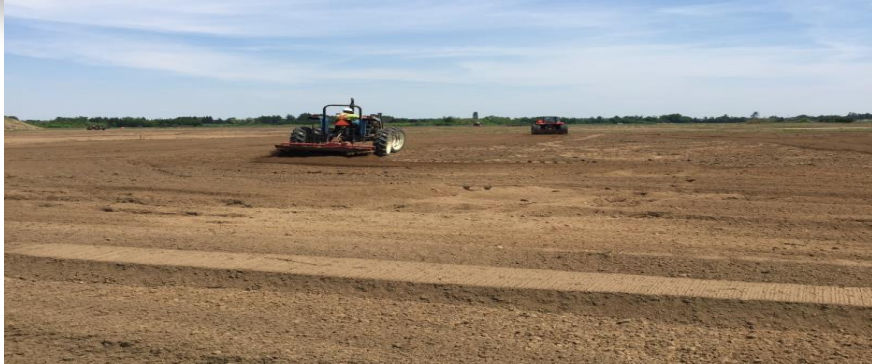
Off-site treatment of excavated soil in mixed biopiles
