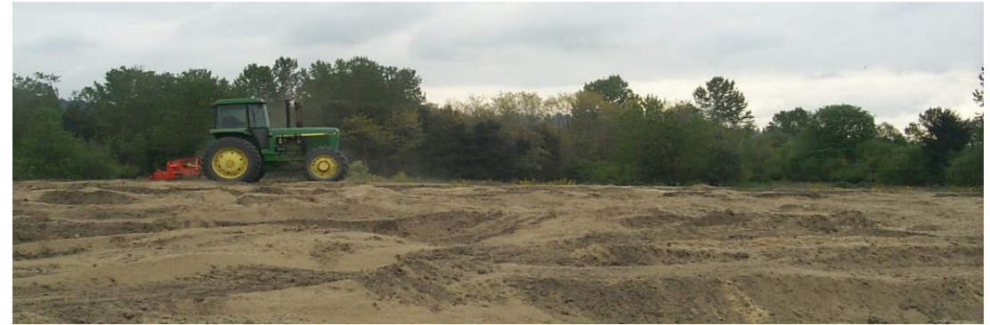
On-site treatment of excavated soil in aerated biopiles
