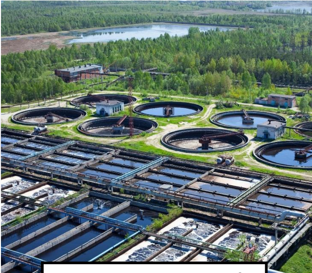
SANI Sewer to Treatment Plant
