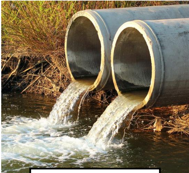
Storm Sewer to River
