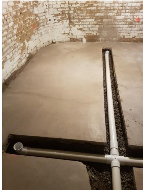
Trenched perforated pipe
