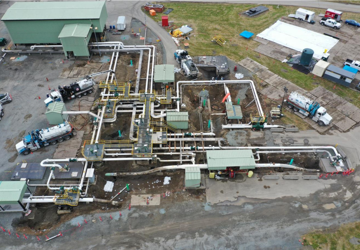
Excavation and product recovery around existing infrastructure
