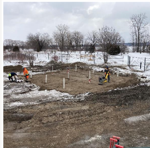
Installing/Compacting of a Low-Permeability Clay Cap
