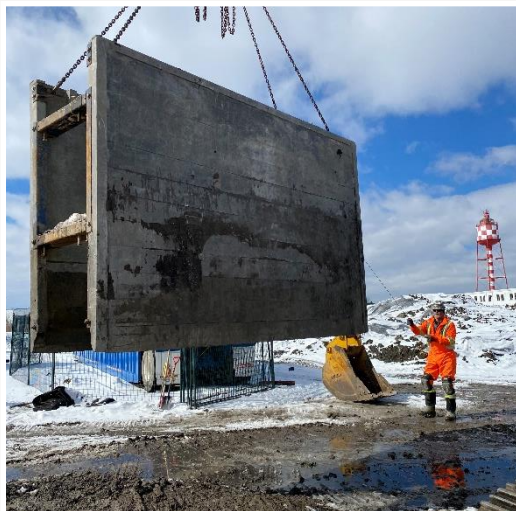
Removing Trench Boxes
