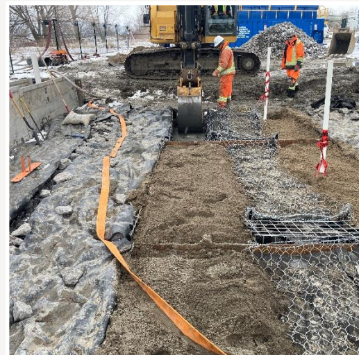
Placing of Adsorption Materials
