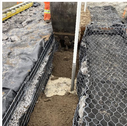
Placing of Pre-Packed Monitoring Wells
