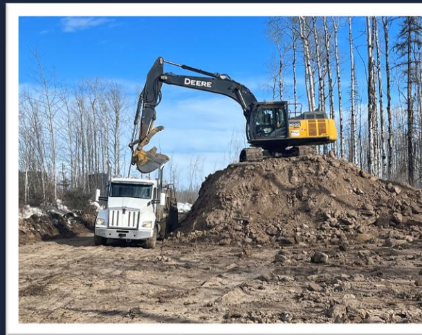
LOADING CLEAN BACKFILL
