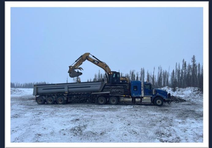
TRUCKING CONTAMINATED SOIL TO LANDFILL
