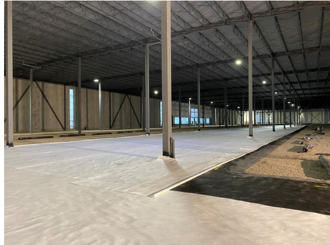
Shield fabric installation
