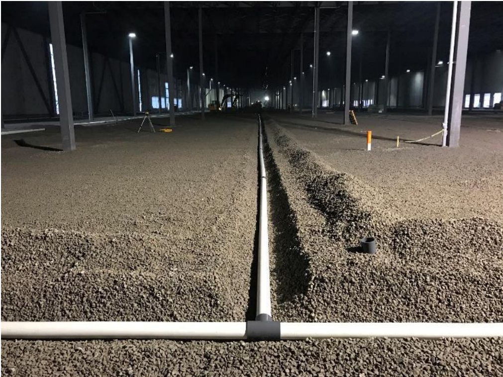
Slotted Pipe Installation
