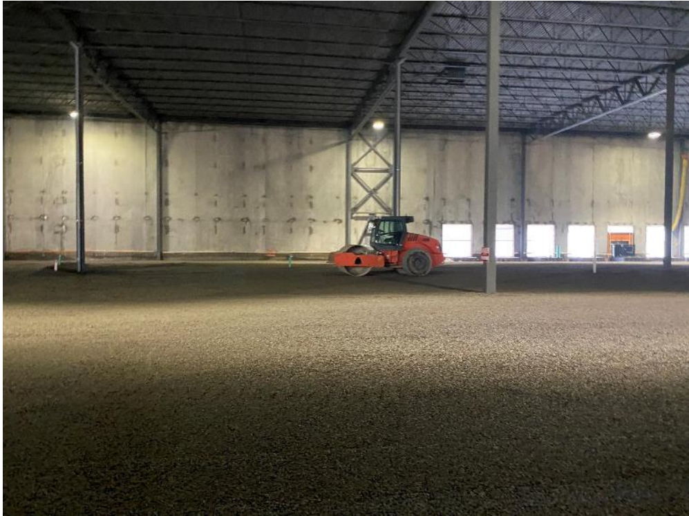
Venting layer compaction
