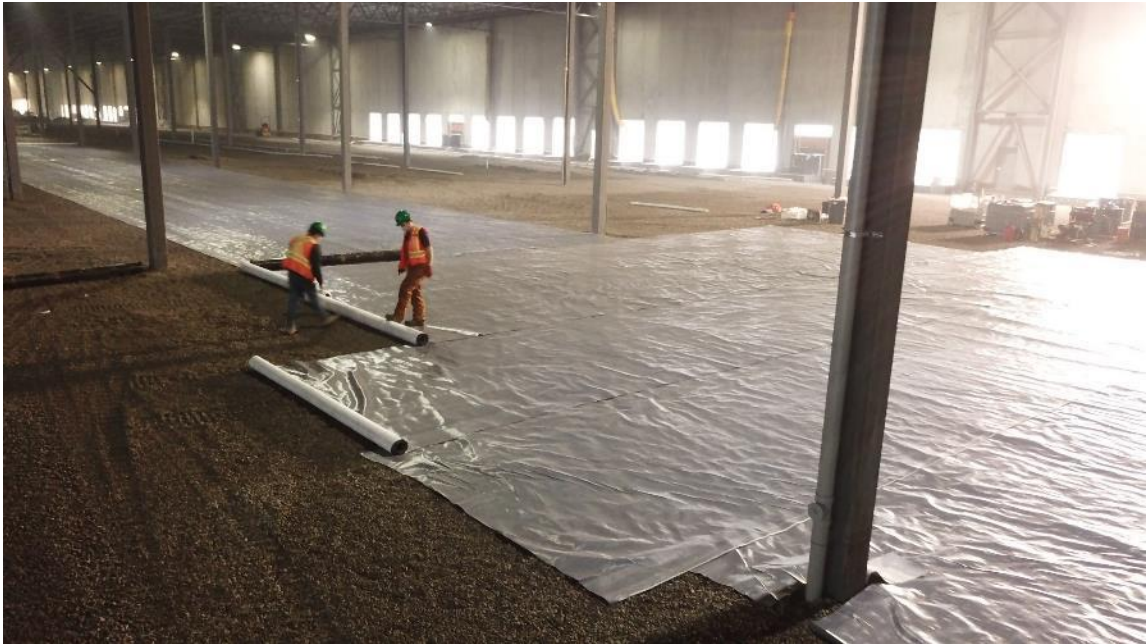
Base Fabric Installation
