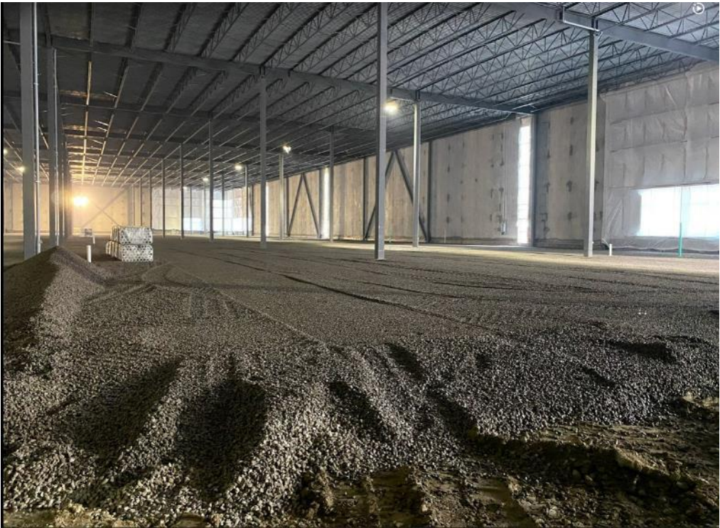
Gravel layer grading
