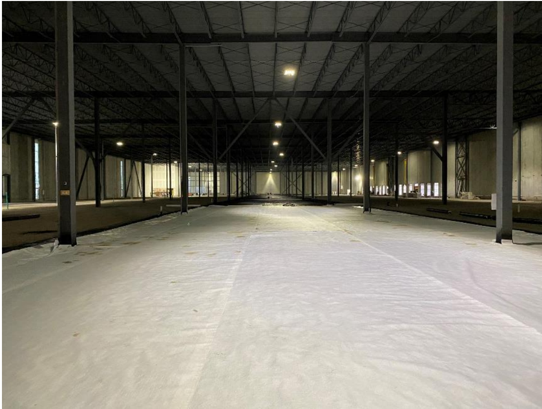
Shield fabric installation
