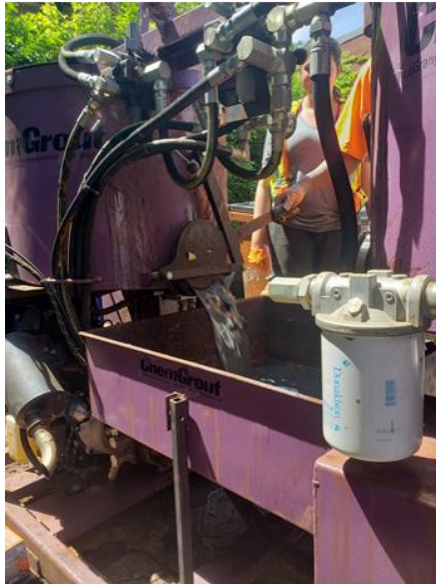
Mixing ZVI Slurry
