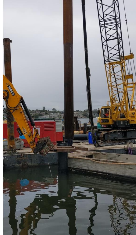
Removal of Buried Piles with a Pile Driver
