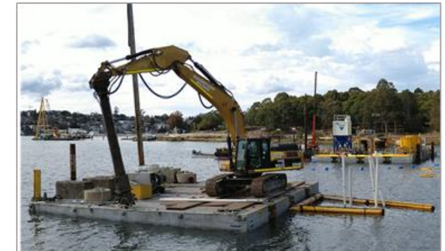
Mass mixing tool to build ISS raft
