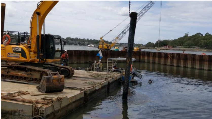
Removal of Buried Piles with an Excavator
