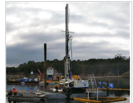
Auger mixing tool to build ISS columns
