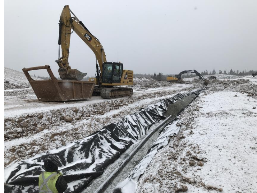
– Interceptor pipeline installation
