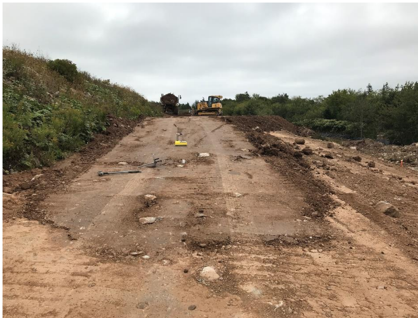
- Compaction testing on berm
