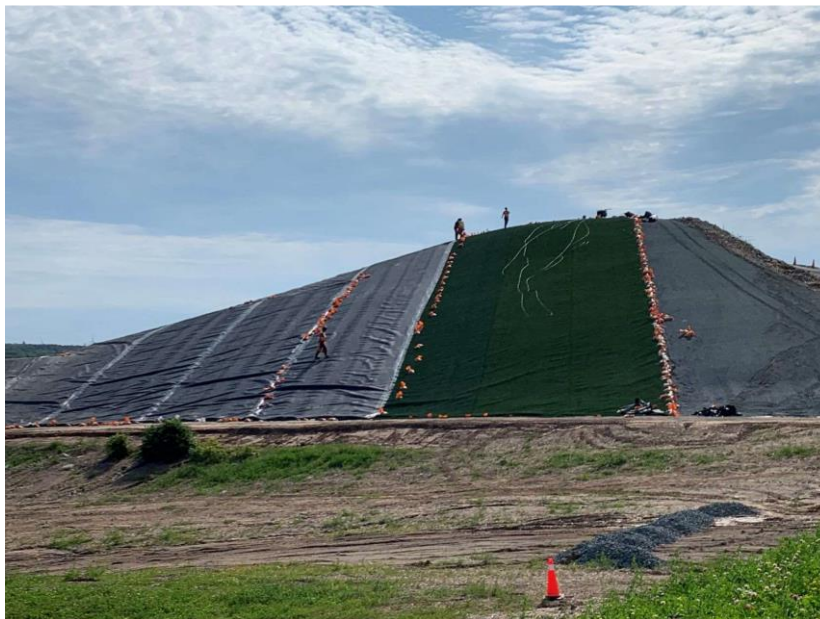
- Liner installation
