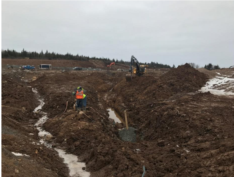
- Trench excavation for interceptor piping
