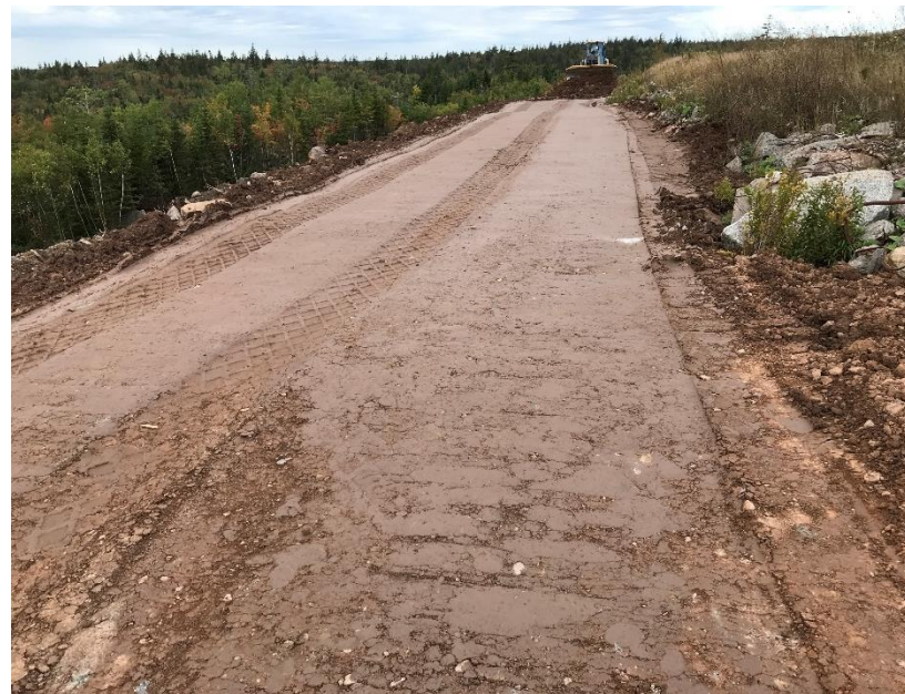
- Construction of perimeter berm
