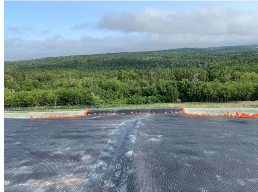
– Micro drain liner installation
