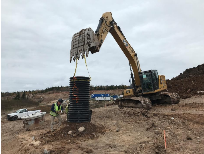
- Landfill sump extension
