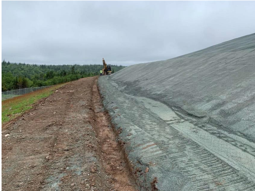
- Anchor trench for liner installation
