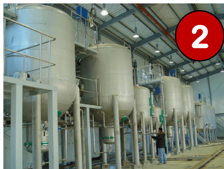
Ex situ Bioreactors (mostly aerobic)
