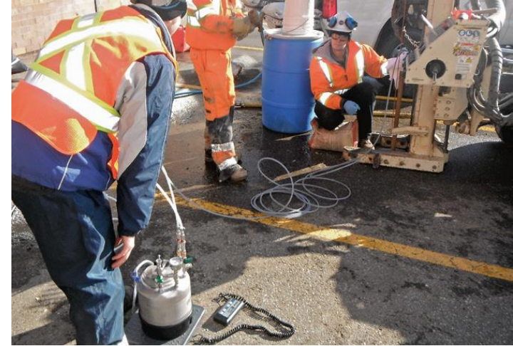
Injection of KB-1 at GTA Site -Photo Courtesy of Terraprobe Inc.
