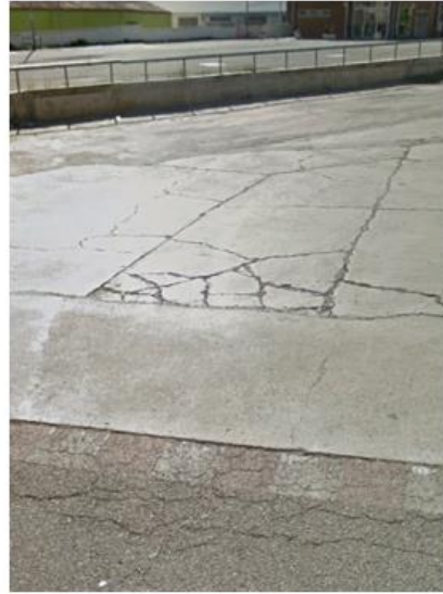
Low diffusivity layer at surface; gas exchange through cracks
