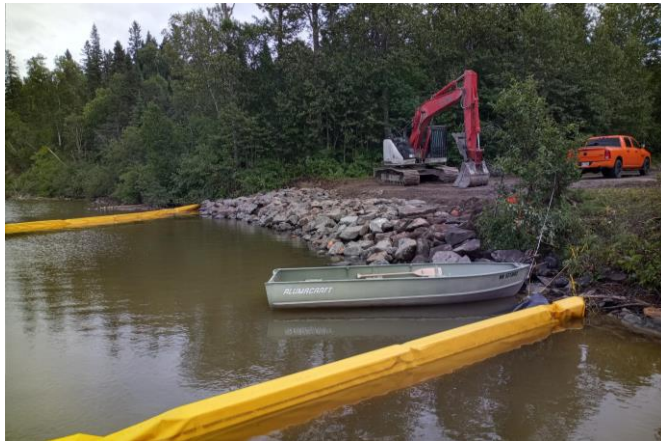
Pic River Bank Stabilization
