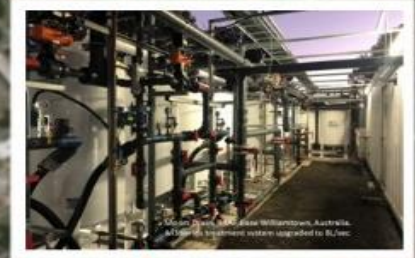
Moors Drain Plant
