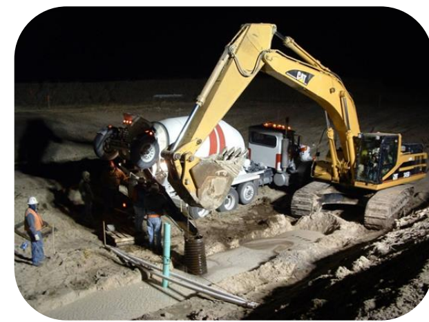
Permeable Reactive Barrier (PRB) – ZVI Cr(VI)
