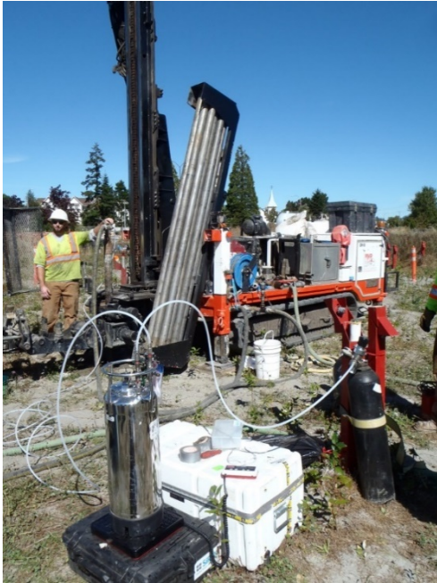
Injection of KB-1 at a site in BC
