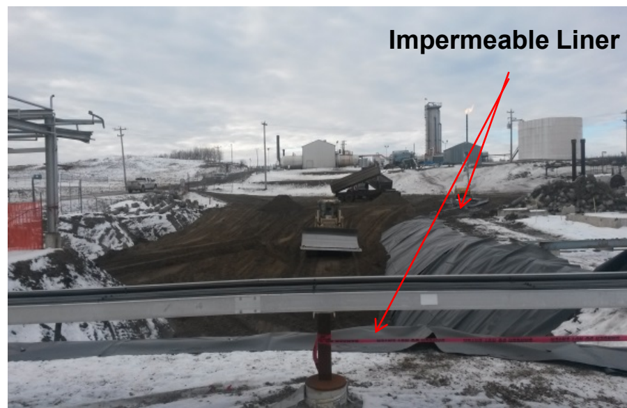
Backfilling activities: west view
