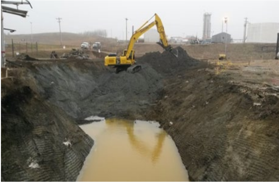
PHC-impacted soil and concrete: Class II landfill disposal
