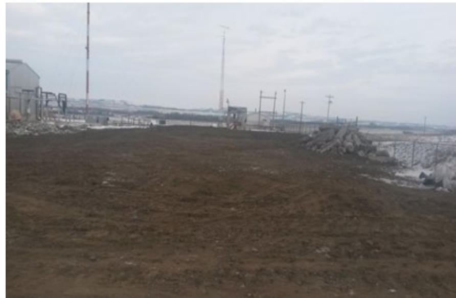
Backfilling activities completed: east view
