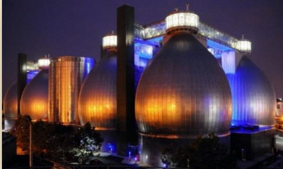
Anaerobic Digesters
