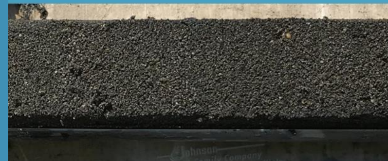
After PetroFix Injection
