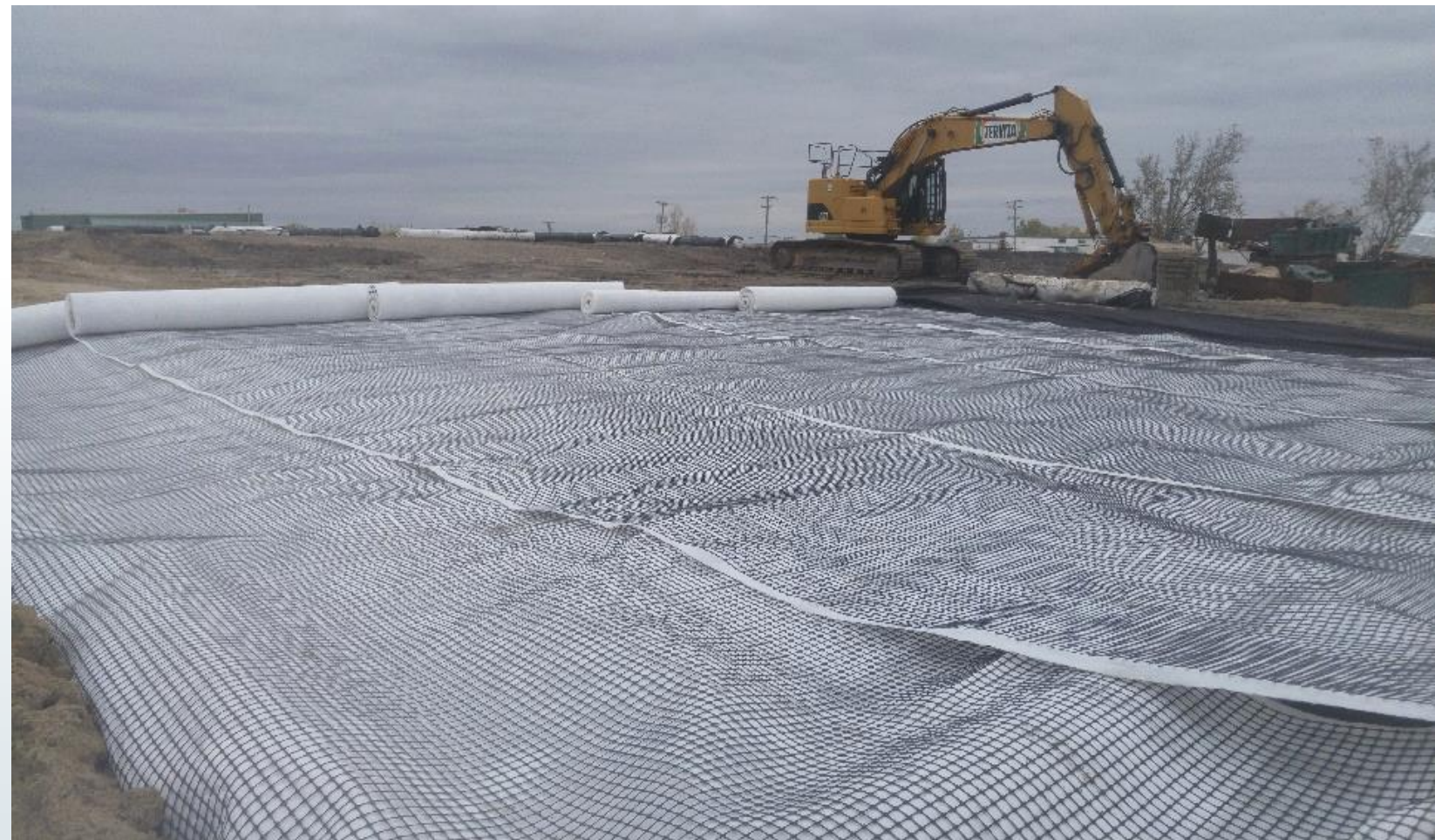
Placement of geogrid on engineered cap and ramp
