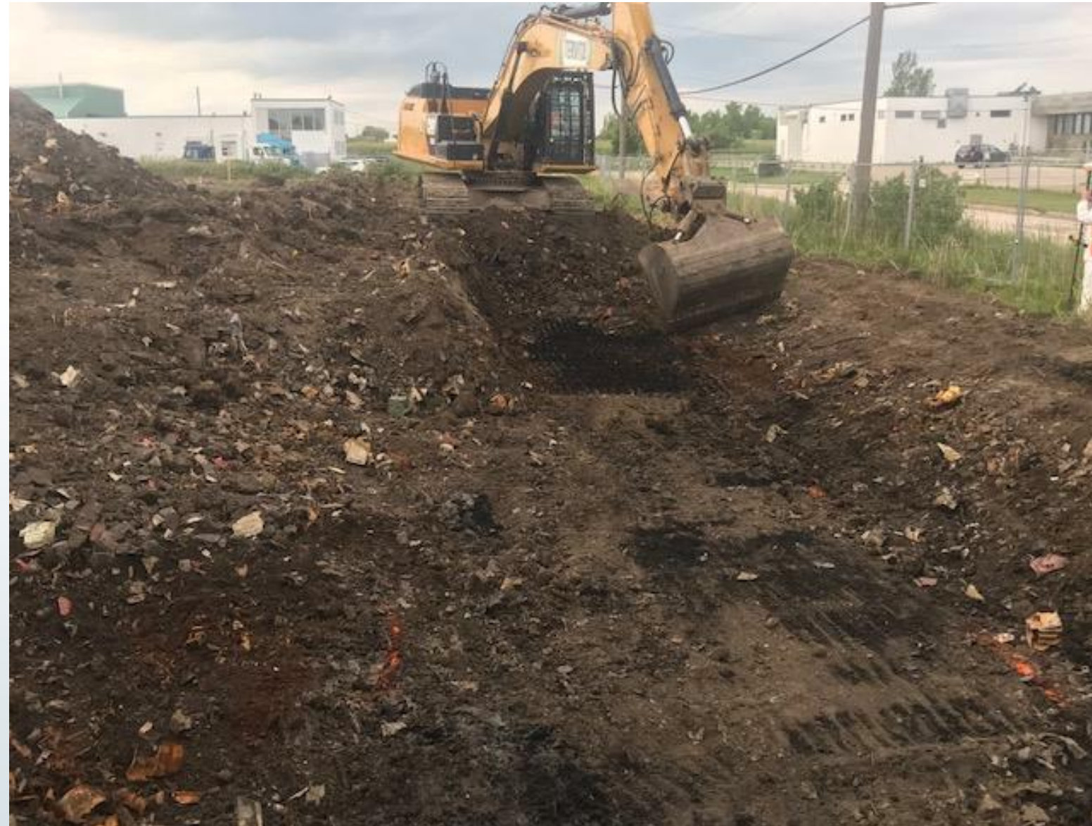
Battery casing debris encountered in northern section of site
