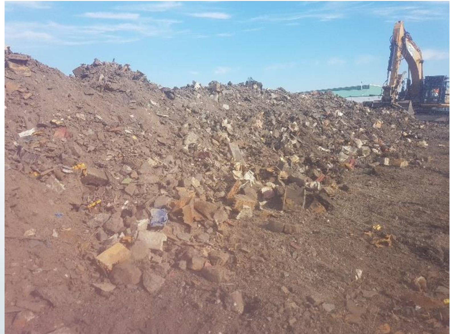
Battery casing debris encountered in northern section of site
