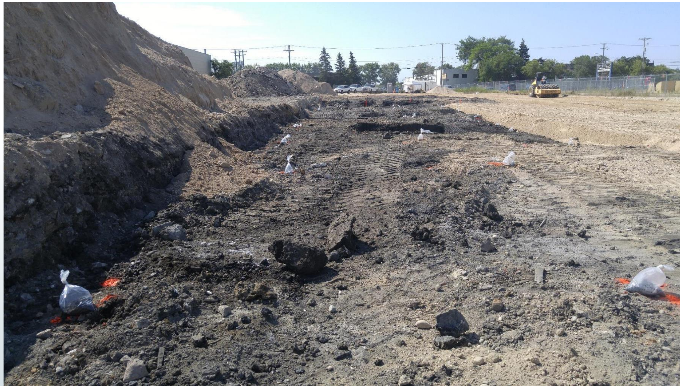
Soil screening in excavation
