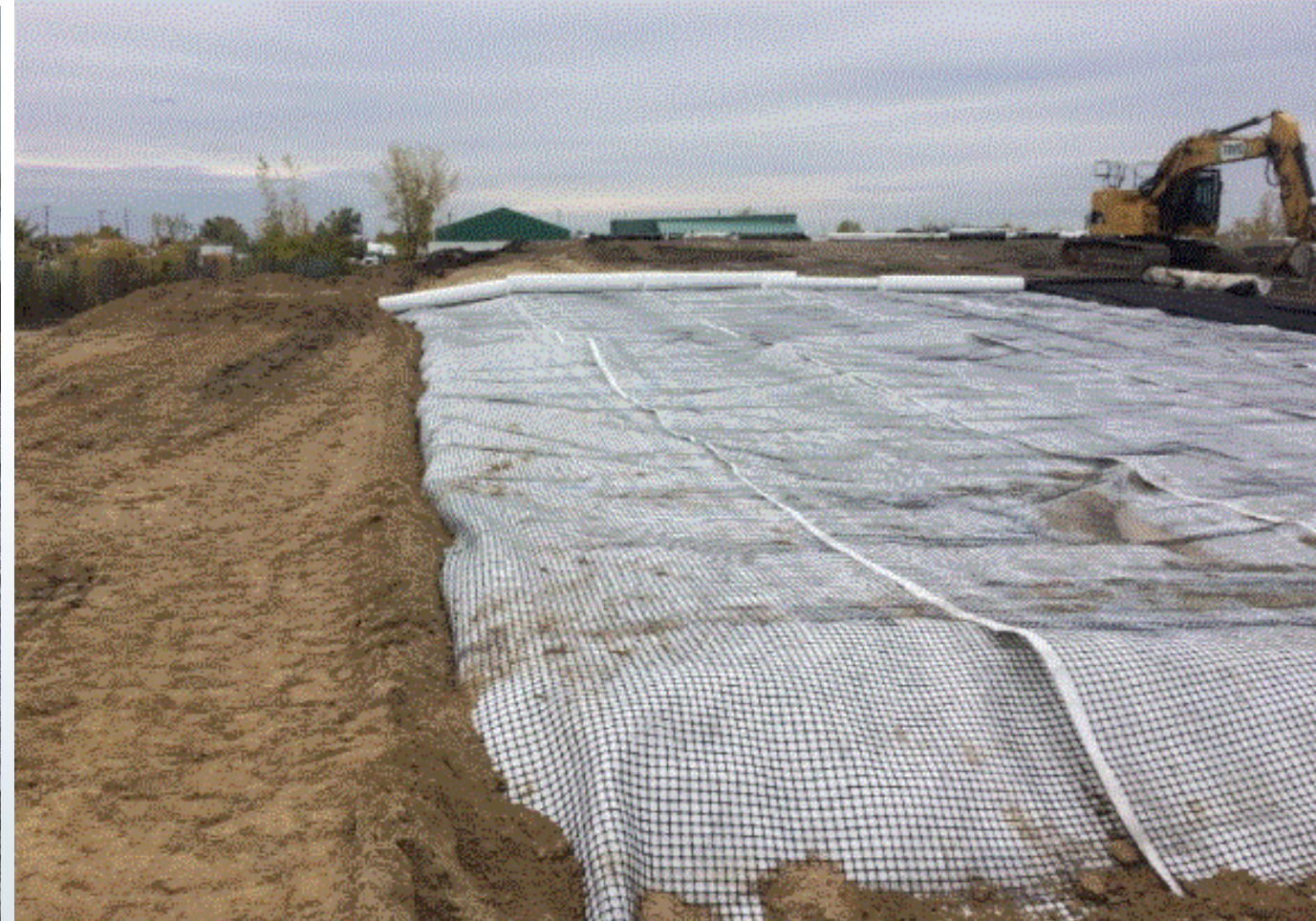
Placement of geogrid on engineered cap and ramp
