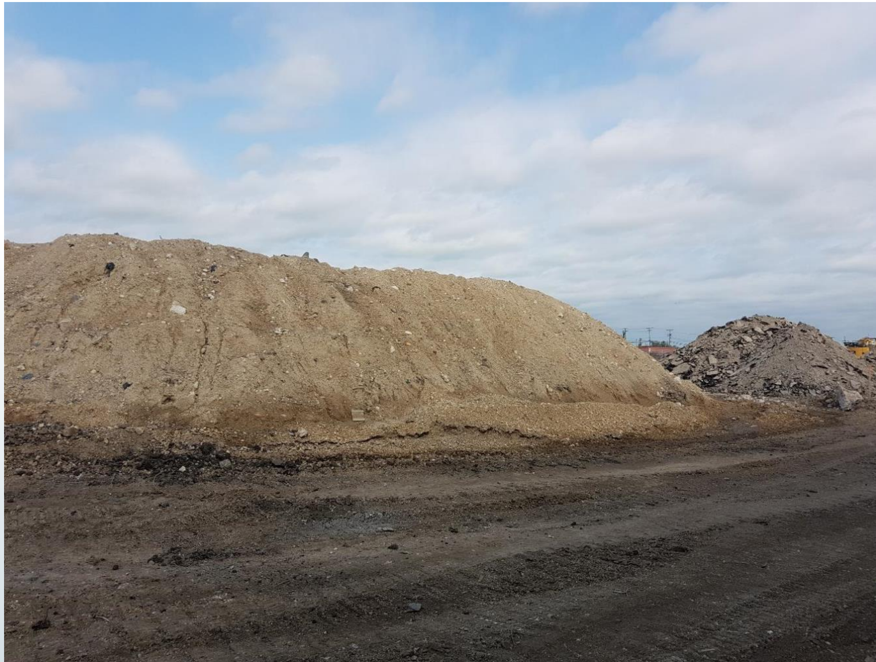
Metal Impacted granular fill material and asphalt
