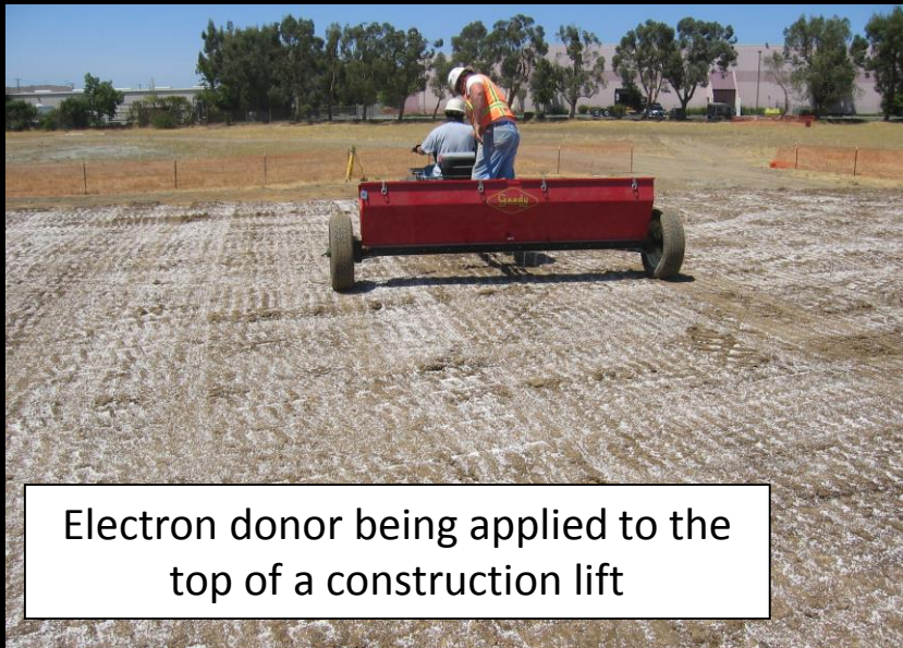
Construction of pile in 15 cm lifts
