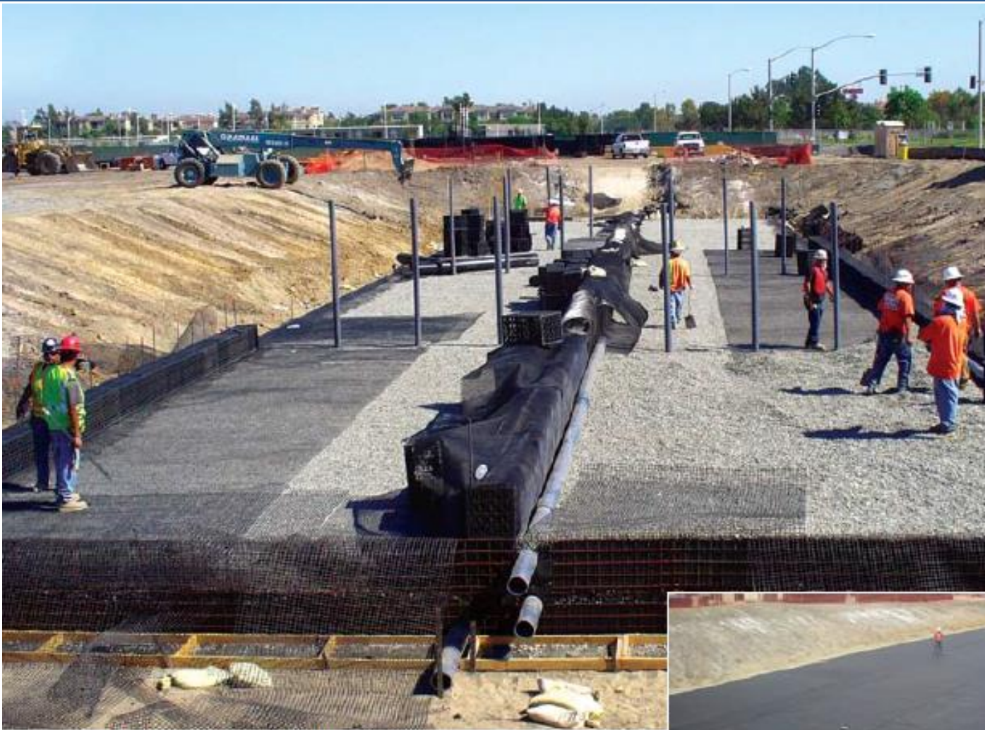
Photo 1 | Construction procedure of the biofilter cell: geomembrane liner installation for the bottom of the cell (inset photo). Startup placement of geogrids and matrix tank modules (above).
