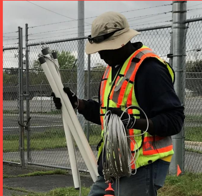
place soil into screened housings
