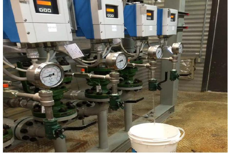
Infiltration Gallery Well Samples Being Collected into a Clean Bucket
