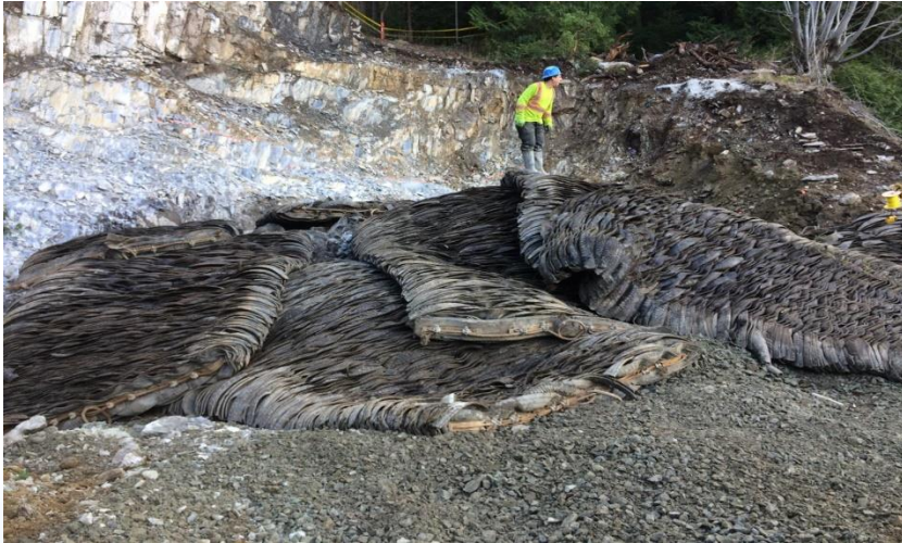
Blast mats installed prior to blasting rock
