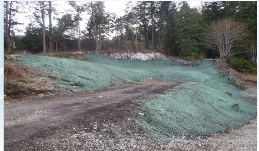
Final layer of hydroseeding
