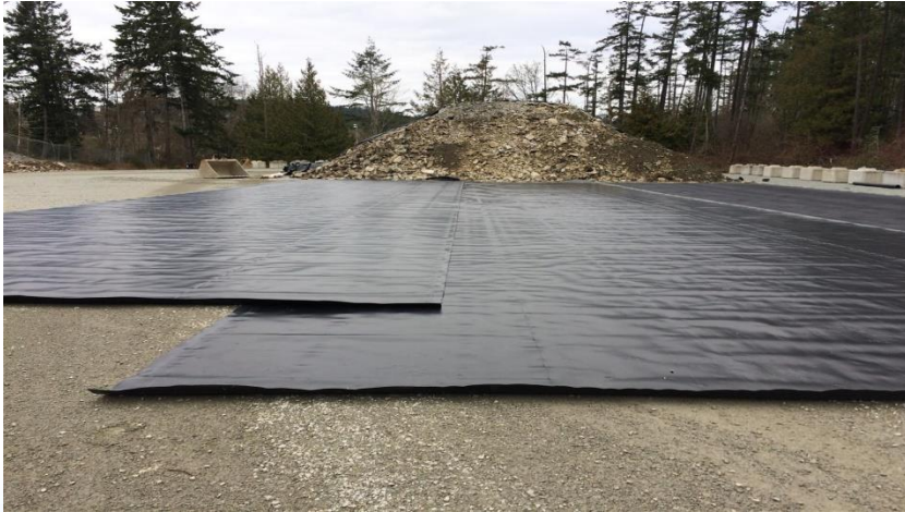
Contaminated waste rock stockpiled on liner
