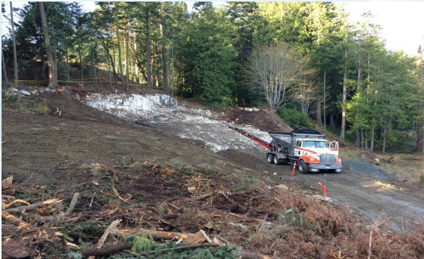
Placement of topsoil over backfilled excavation
