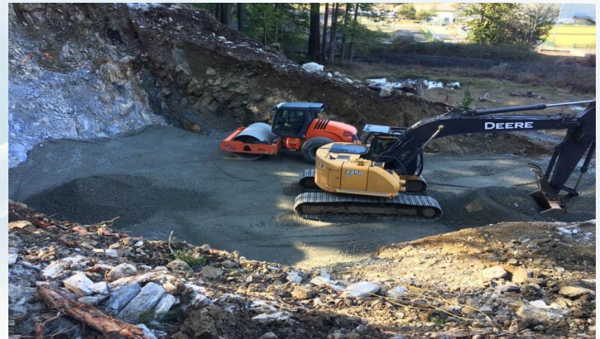
Clean backfilled excavation floor
