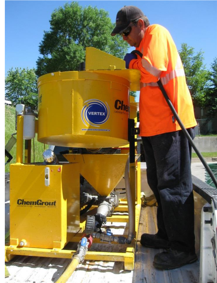
Mixing ZVI slurry for injection
