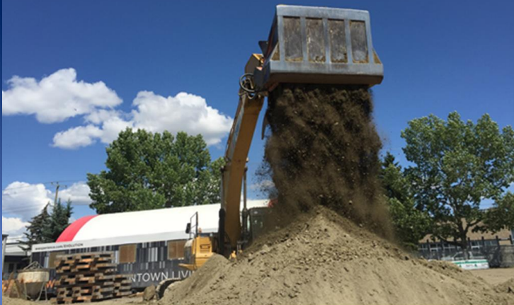
Allu bucketing Class I soils Prior to Treatment
