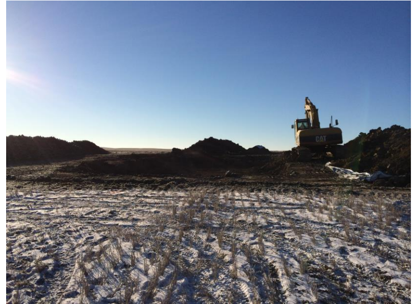
Single windrows, stripped to edge of a large work area, accommodate recontouring uniform replacement.
