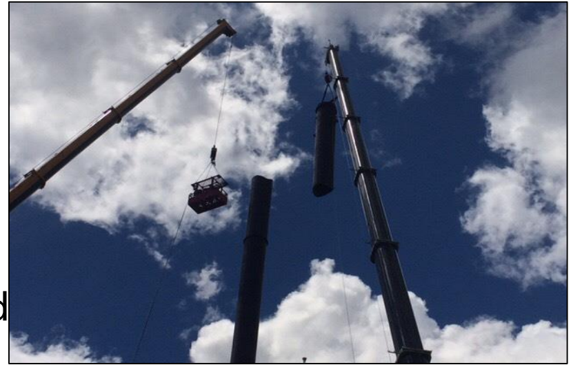
Critical Lift – Stack Removal
