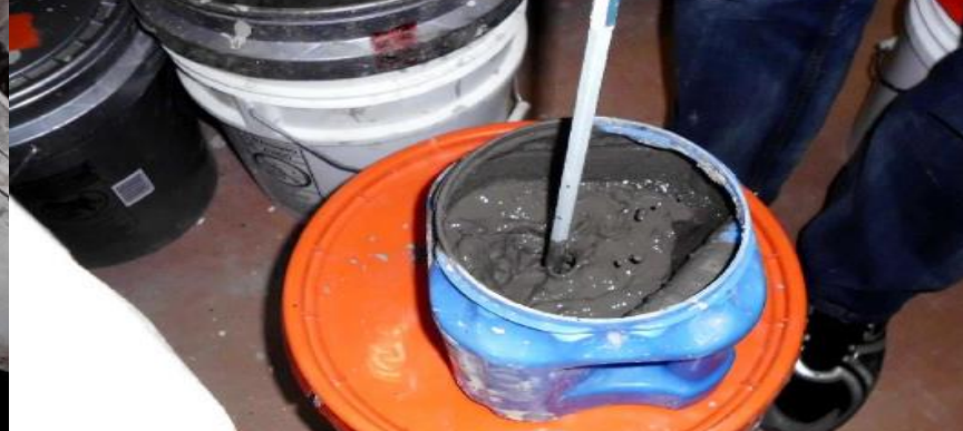
Add grout to achieve workable material
