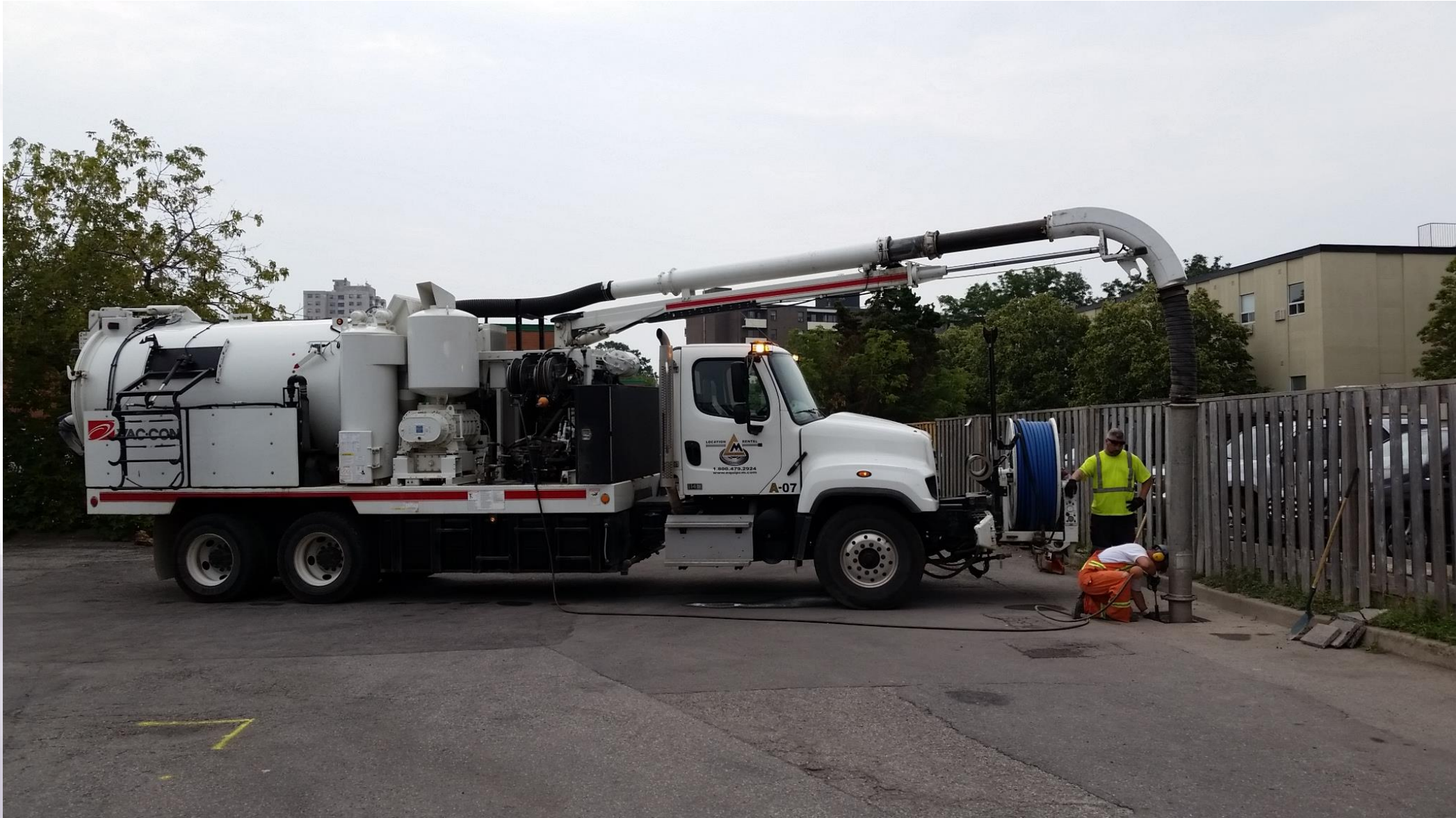
Hydro-vac'ing Top of Sewer
