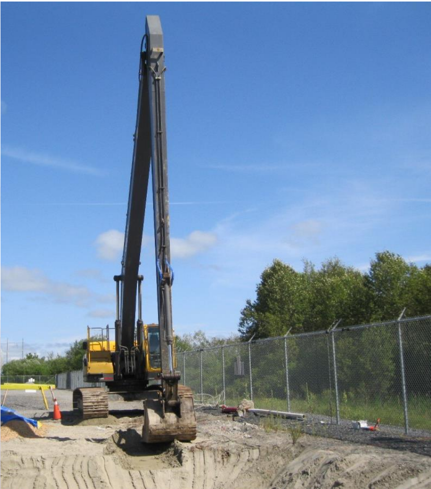
Potassium Persulphate Soil Mixing PRB
