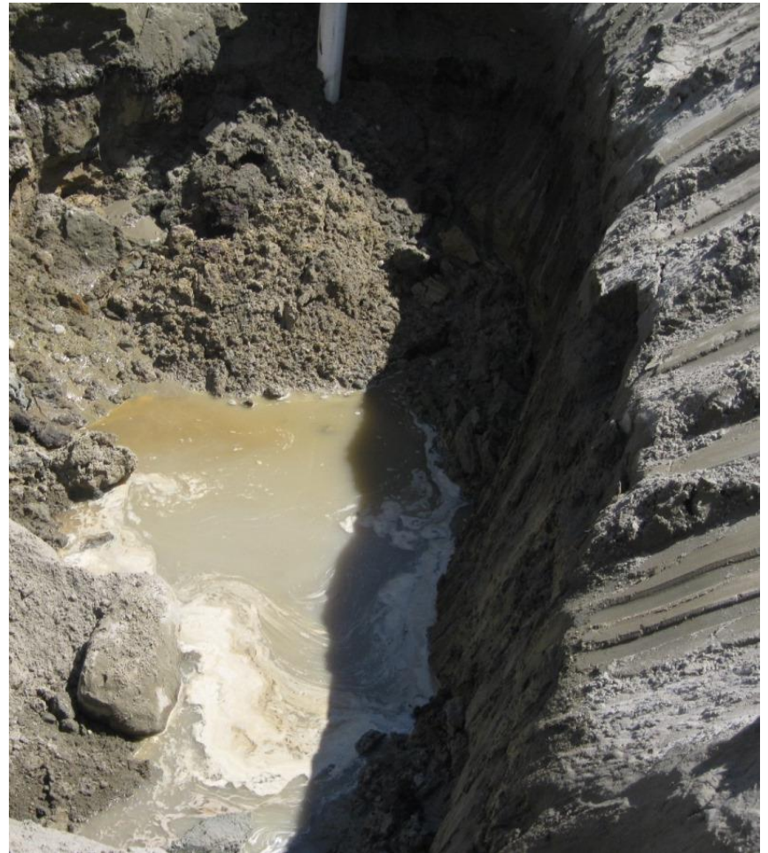
Potassium Persulphate Soil Mixing PRB
