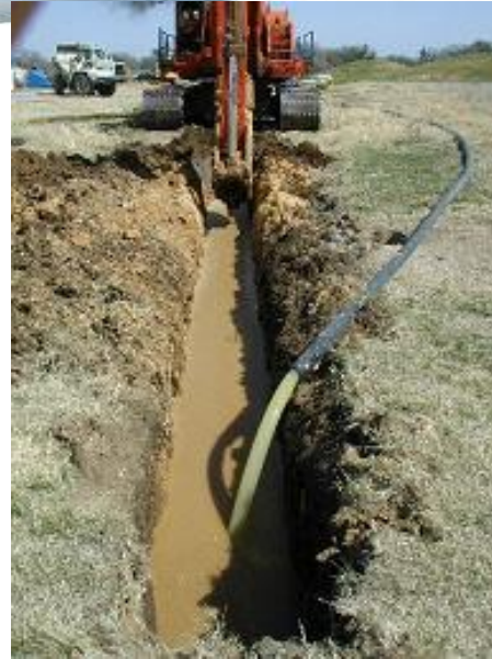
biopolymer trenching (70 ft, 21 m)
