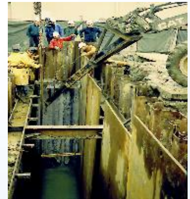
Cofferdam/trench box (30 ft, 9 m)
