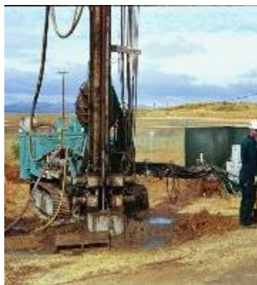
jetting techniques (60 ft, 18 m)
