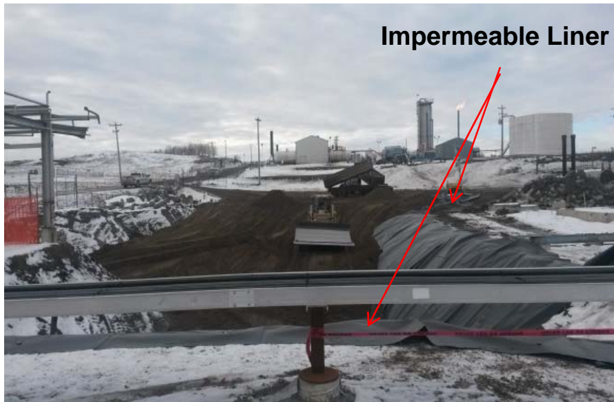
Backfilling activities – west view
