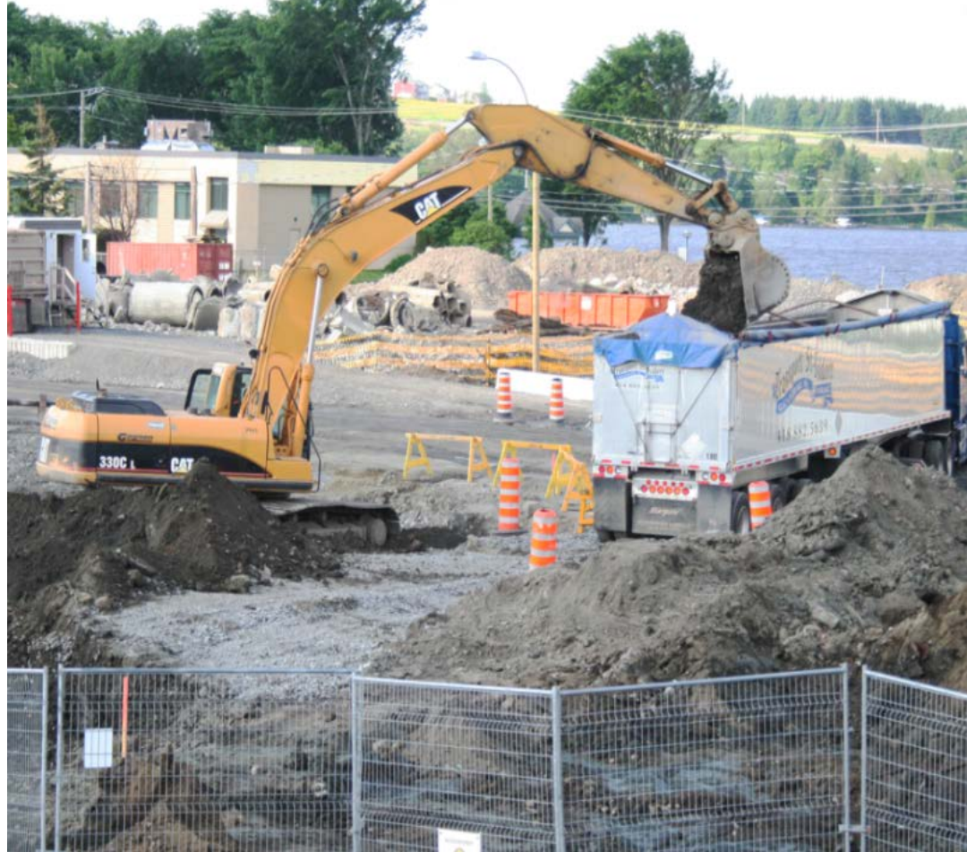
Impacted soil being loaded for treatment/disposal; Lac Mégantic visible in background
