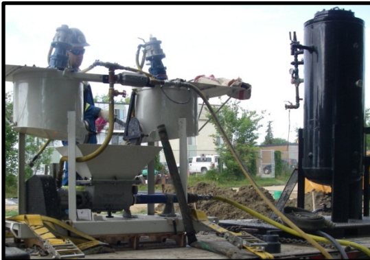
Filter Sand and Grout Equipment
