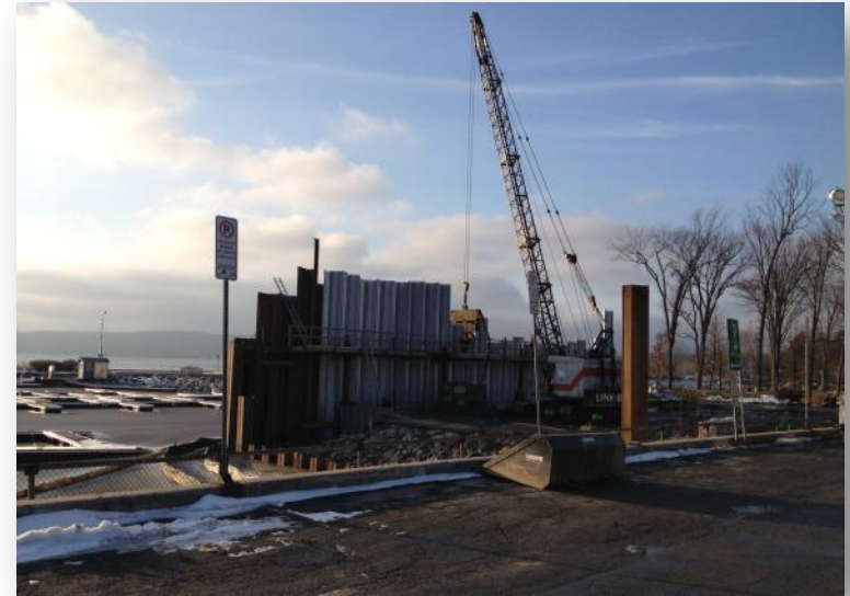
Installation of sheet piling
