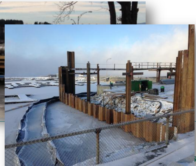
Installation of sheet piling
