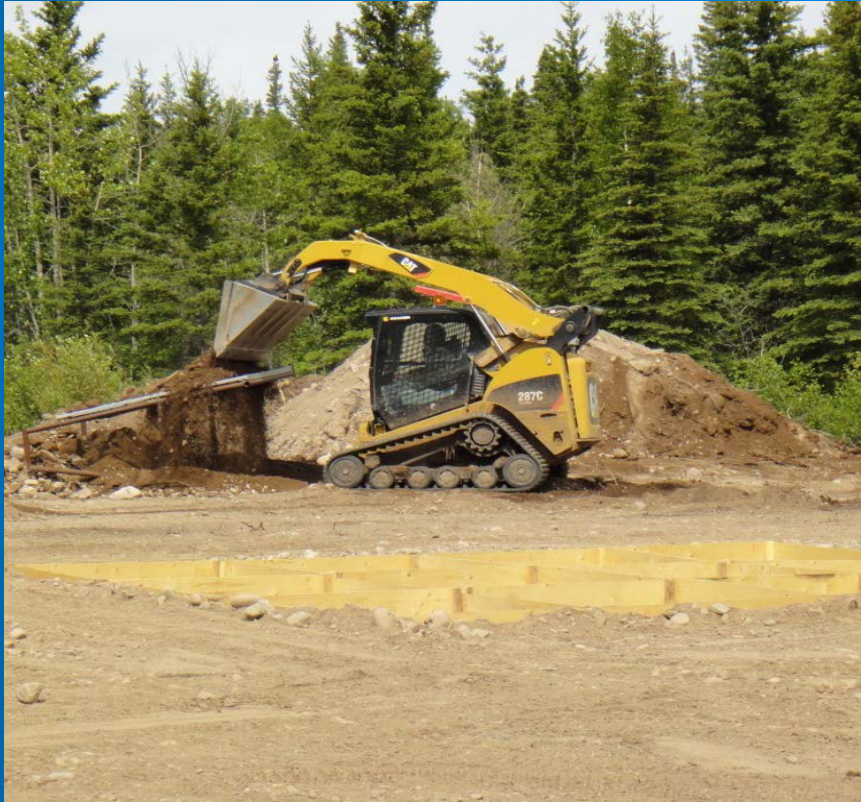
Borrow material screening
