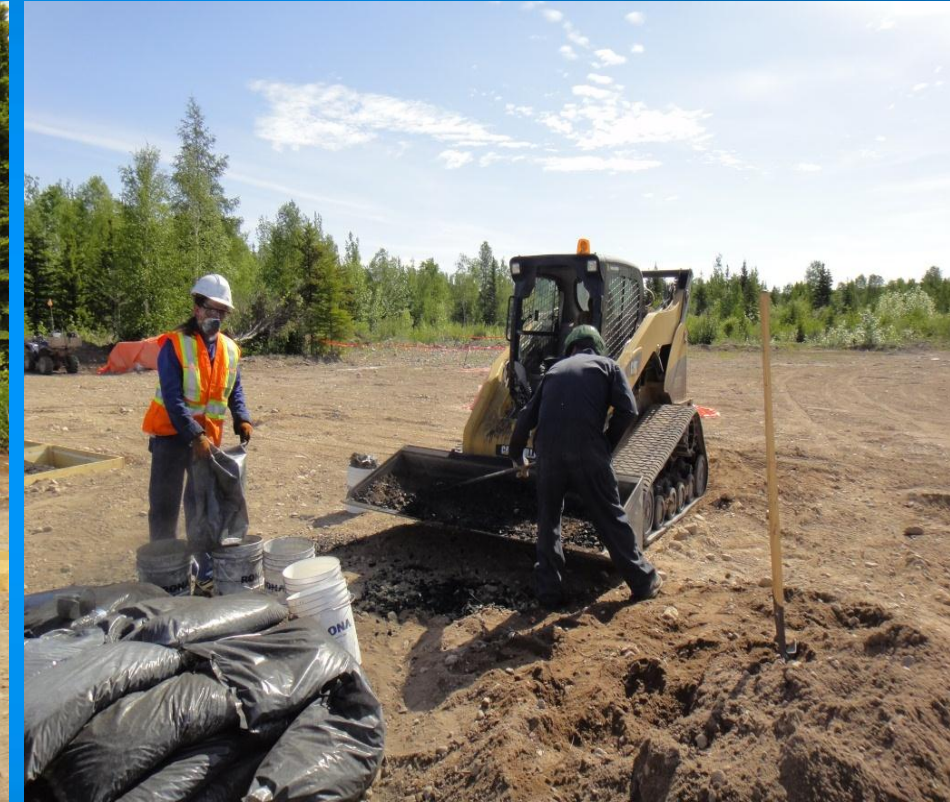
Preparation of the soil mixture from borrow material and biochar
