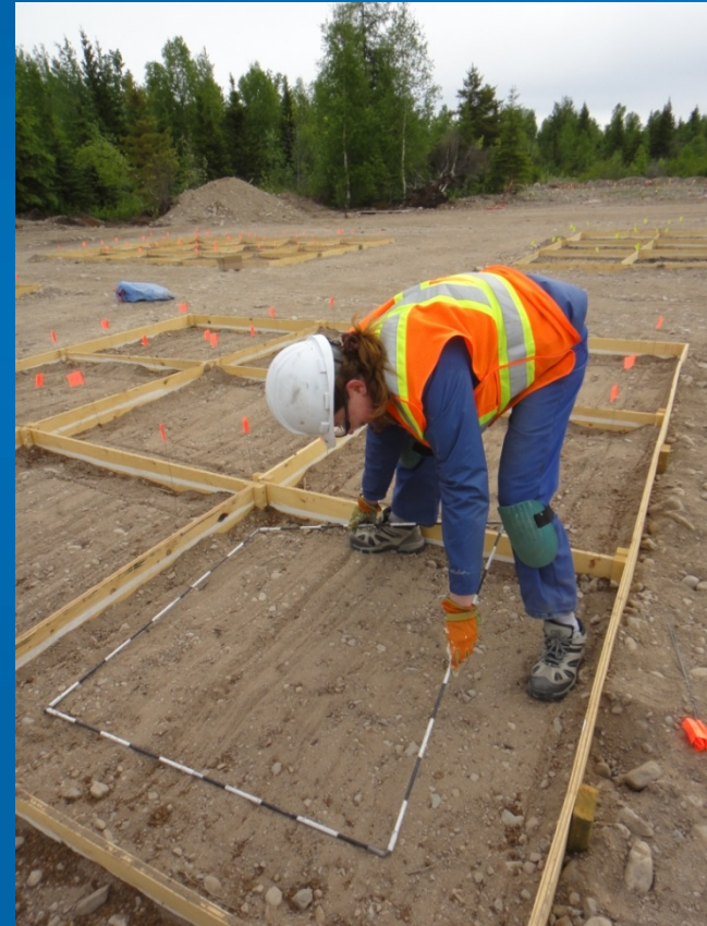
1m 2 frame installation
