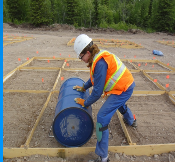
Soil compaction
