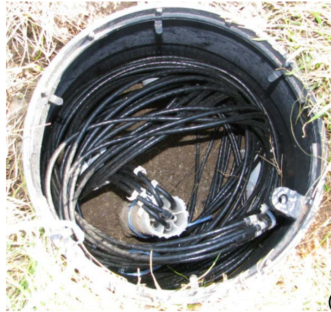
CMT system for monitoring
