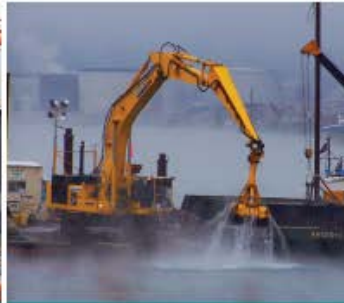
Dredging & Sediment Remediation
