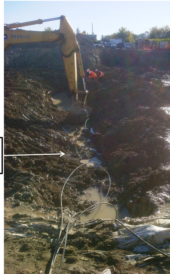
Installing HWs into Excavation
