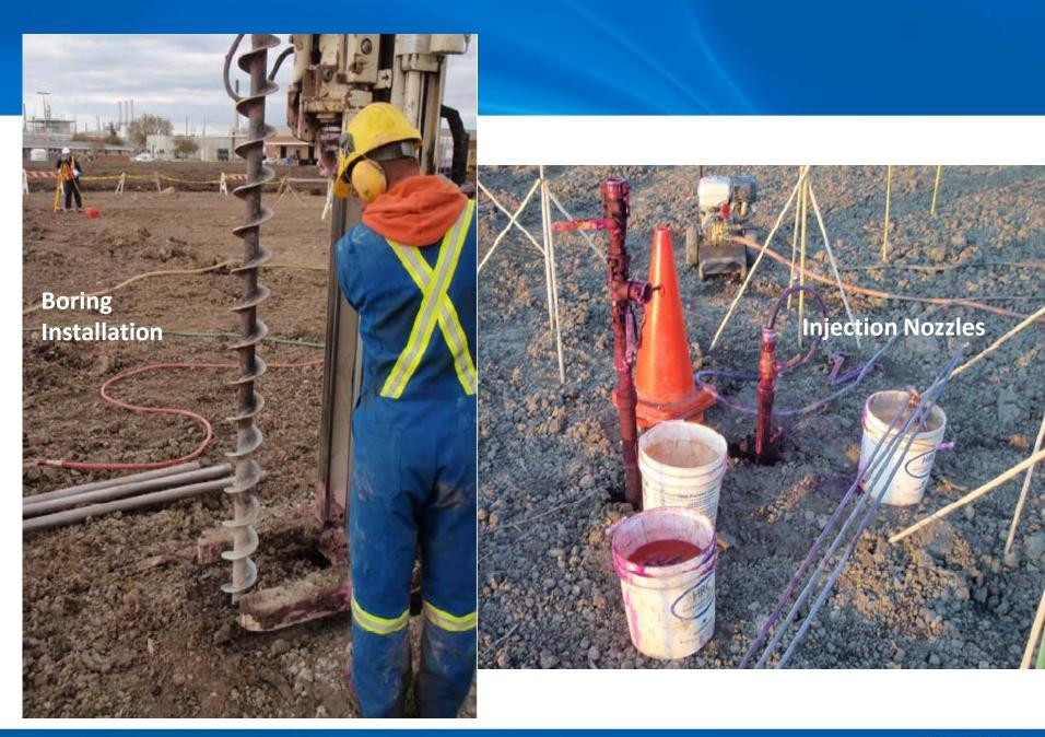
Each location had 3 fracture depths, each finished with a 1" PVC temporary well
