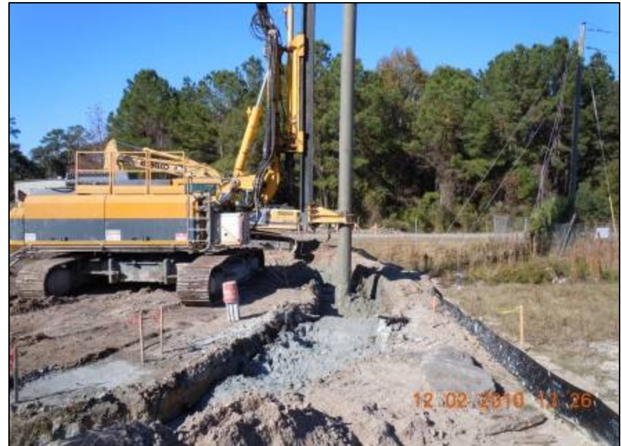
Installing Vertical Wall With A Panel Cutter
