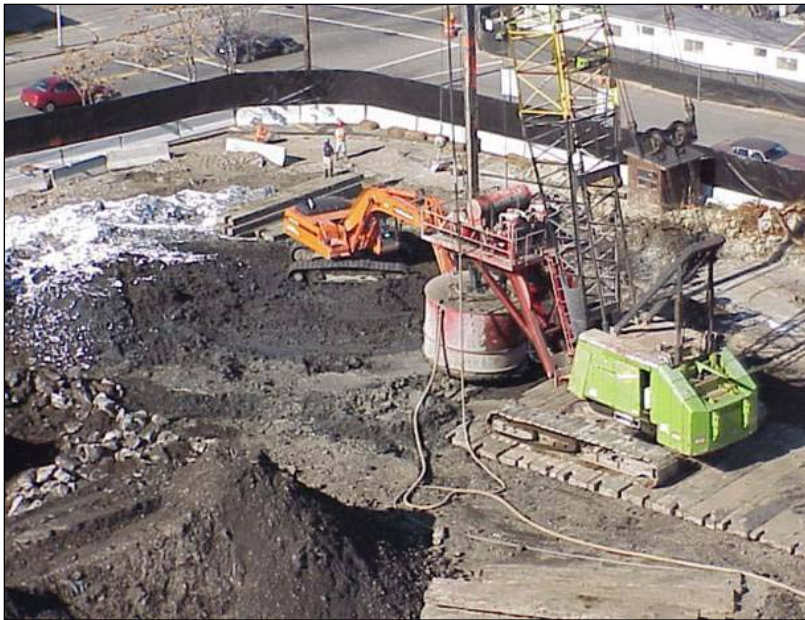
Auger-mixed in situ S/S treatment of a former manufactured gas plant (MGP) site with coal tar contaminants at Kendall Square, Cambridge, MA, United States.
