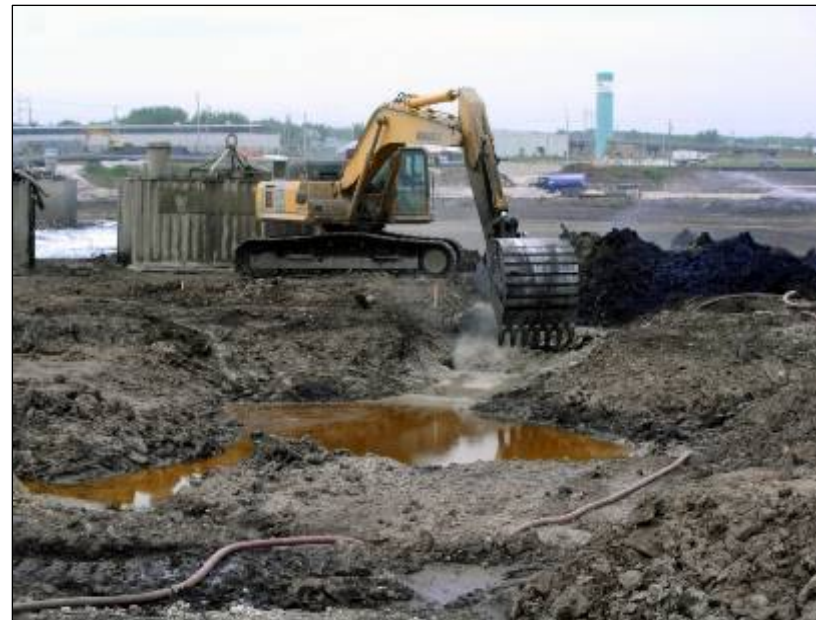
Excavator bucket mixing of contaminated sediment of a former steel mill operation, Sydney Tar Ponds, Sydney, NS, Canada.
