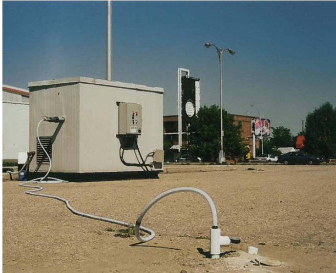
Pilot test equipment set-up. Test well (MW00-16A) in foreground.
