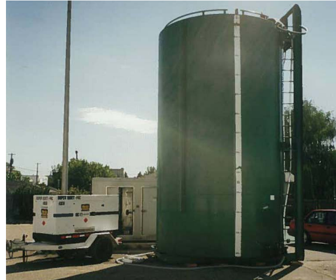
Temporary water storage tank.
