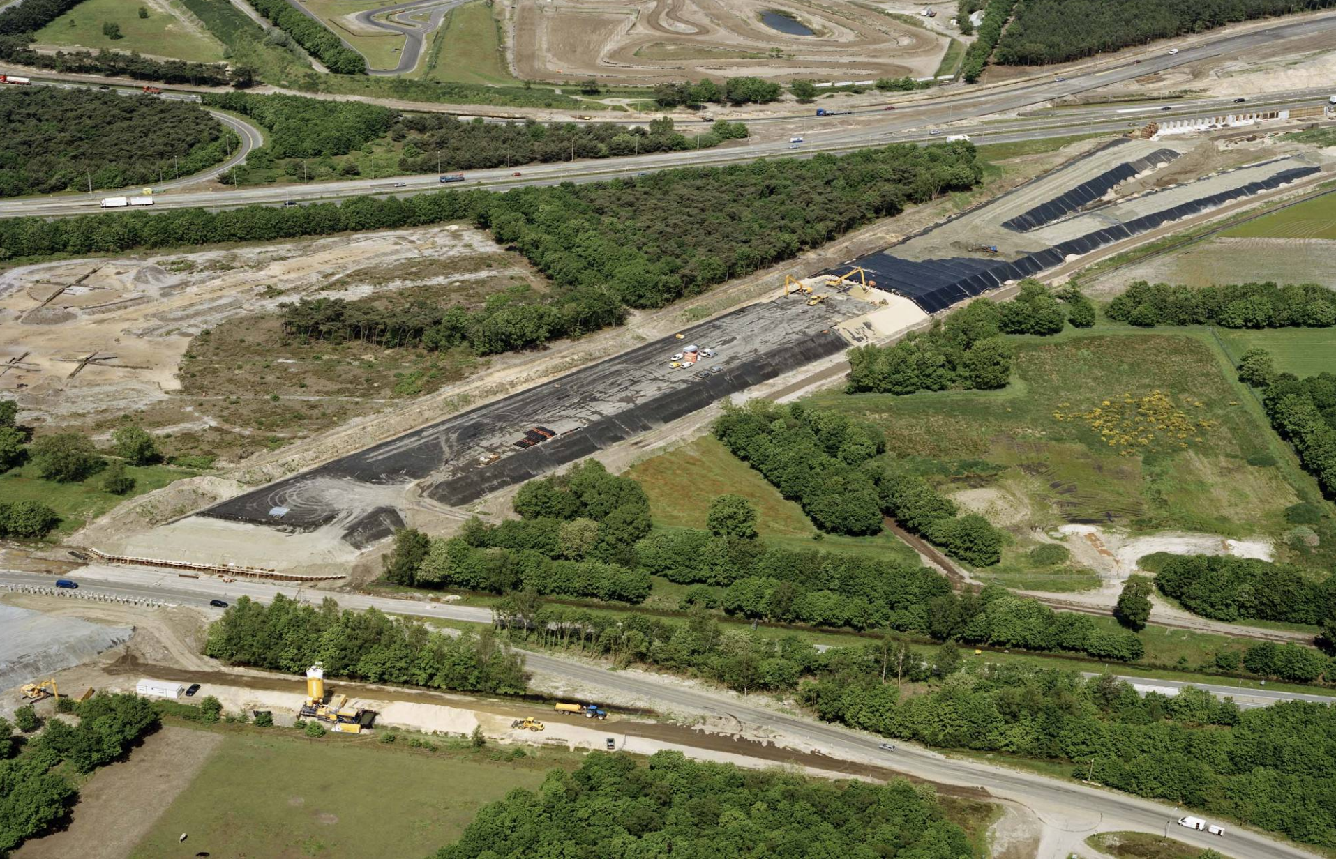
Highway construction Oss Paalgraven, Netherlands 2005-2006
