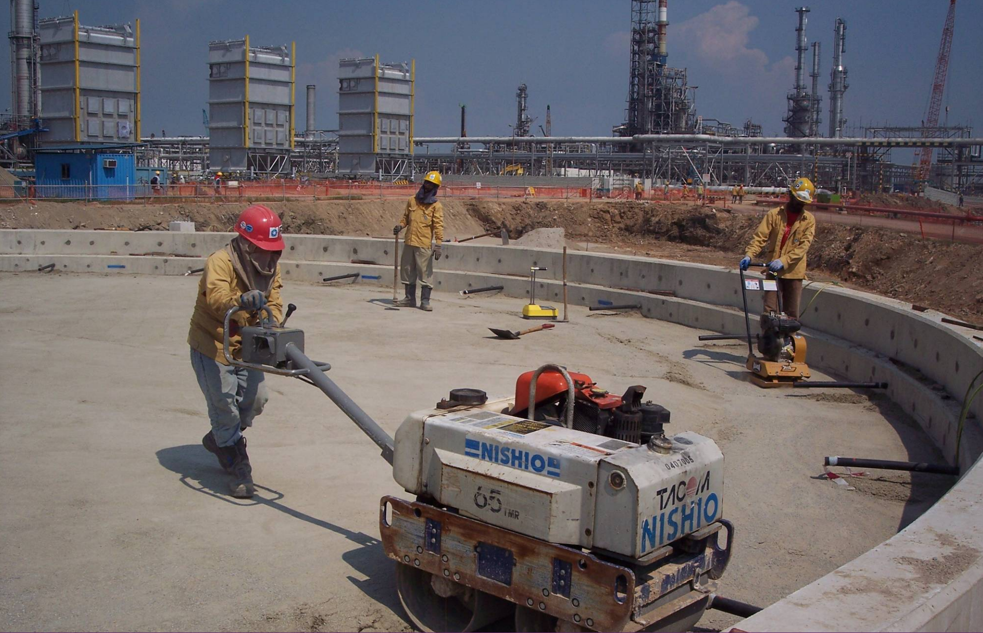
Liner for (benzene) tank park Shell Singapore 2008
